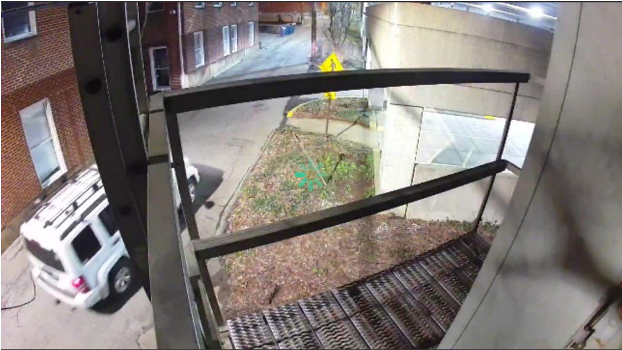
After New Lighting Installed
